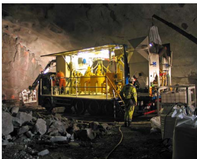
Figure 4. High pressure pre-grouting with modern grouting rig.
